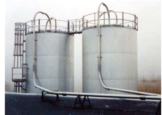
Tank & vessel construction
